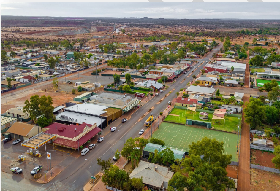
Aerial view of Leonora township
