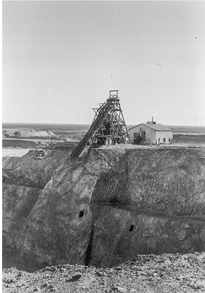
Figure 32 Headframe on the edge of the pit, 1980. Courtesy Shire of Leonora.
