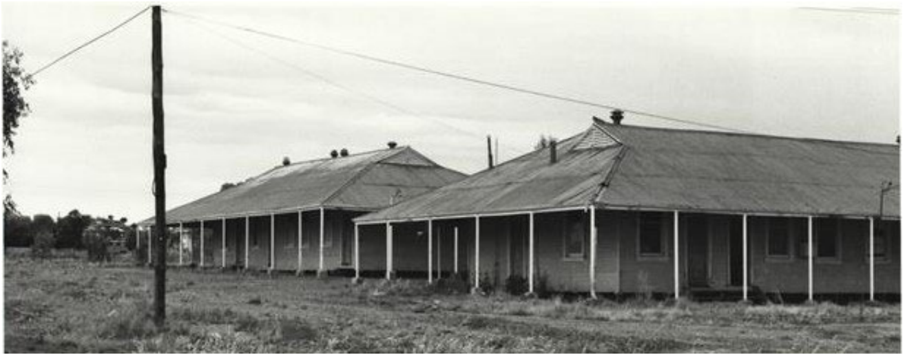
Court House and Mine Office, 1982. Courtesy Heritage Council of WA.
