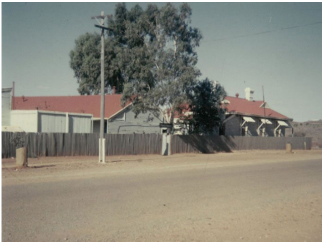
Police Station Group 1962. Courtesy Shire of Leonora.
