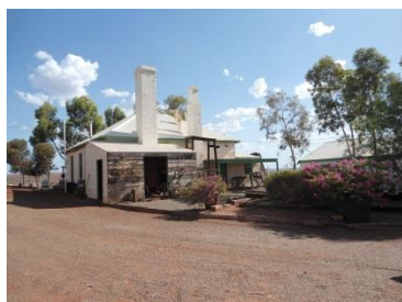
Exterior view of Archive in the Old Assay Office
