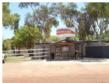
External view of Leonora Lodge
