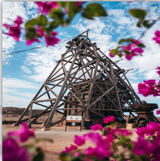
Gwalia headframe — heritage and identity of the Leonora district
